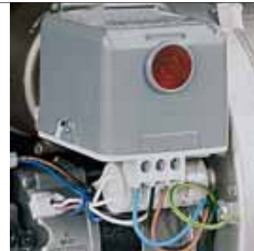
Control box fitted with an ignition transformer
