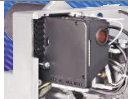
Appliance fitted with an ignition transformer
