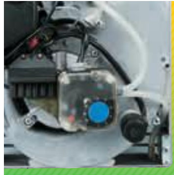
Air pressure switch
